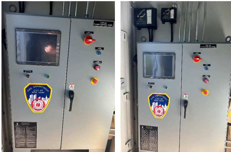
Main Control Panel / Hardware w/ 15" Touchpanel
