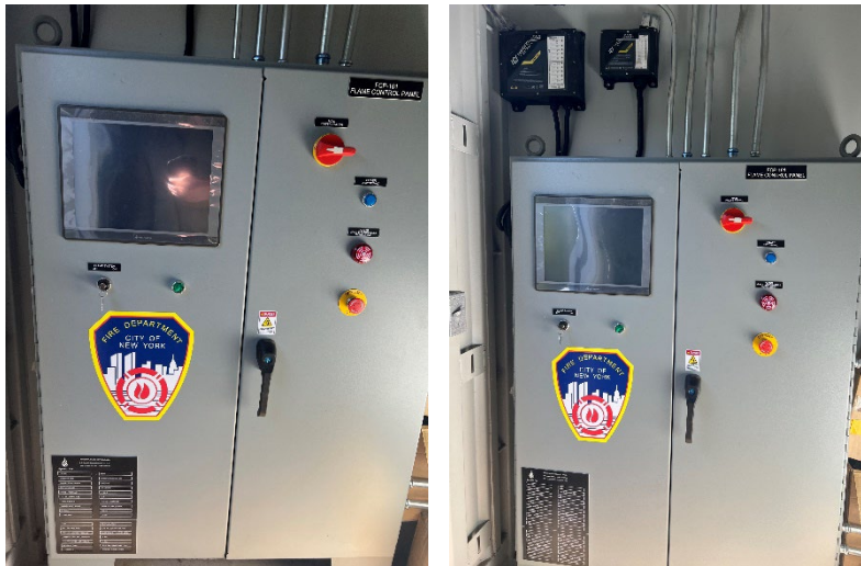
Main Control Panel / Hardware w/ 15" Touchpanel
