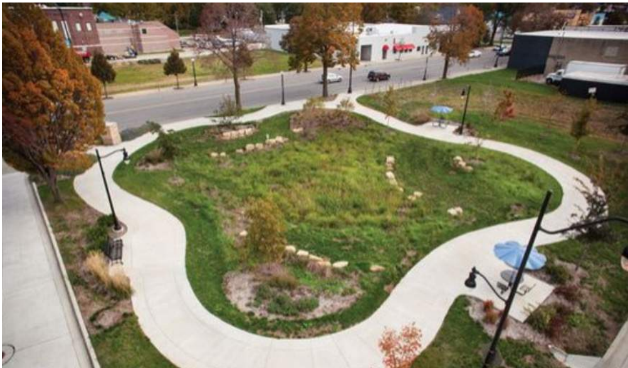
Image 1 - Detention pond garden space
